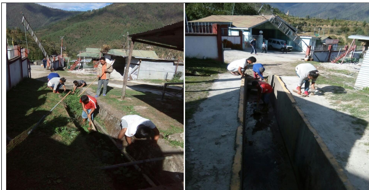
Cleaning of drains of office campus near Feed Technology Unit
