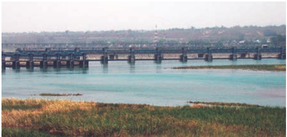
Fig. 2 Madhopur Barrage on Ravi river
