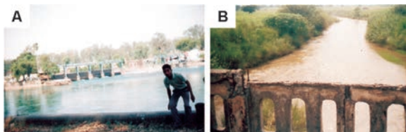
Fig.5 (A) Diversion of water from Madhupur into UBDC and Hydel Canal, (B) Ravi-Beas link Canal
