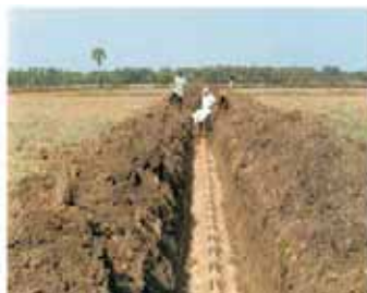
Stoneware pipe collector line packing with sand envelope at coir filled joints
