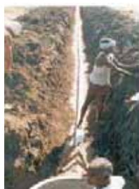
Installation of CPVC collector line with Nylon mesh
