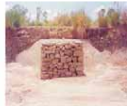
Deflecting Spur with Proper Anchoring
