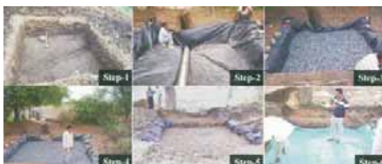
Installation of Type-I recharge filter unit
