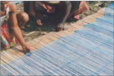
Lining of bamboo screen
