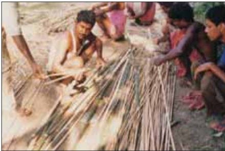
Construction of a bamboo screen
