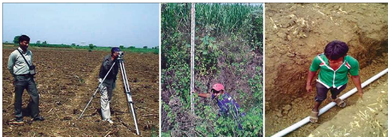
Fig. 1. Installation of sub-surface drainage
