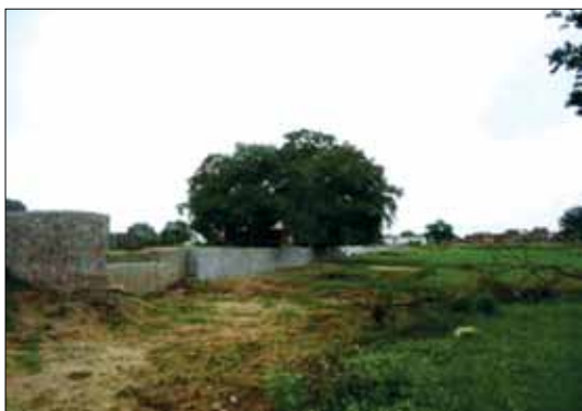
Haveli renovation in Parasai-Sindh watershed; Masonry drop spillway (rectangular weir) and embankment along with corewall was constructed in 50 m breached area. Water harvested in Haveli during the monsoon period. Source: ICAR-Central Agroforestry Research Institute, Jhansi
