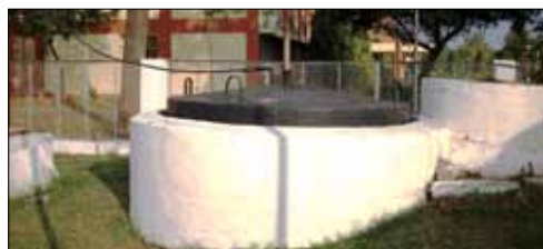
Pile foundation based structurally modified floating drum type bio-gas plant for vertisols.
