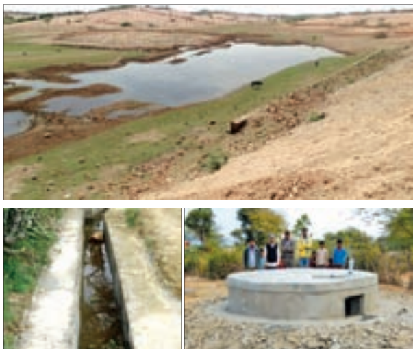
Rainwater harvesting structures in watershed area
